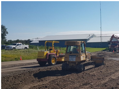
GRADING Parking Lot, Roadways, Gravel Driveways; Excavation, Landscaping, Hired Equipment
