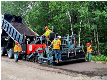
ASPHALT PAVING Pot Hole Repairs, Driveway Paving, Parking Lots
