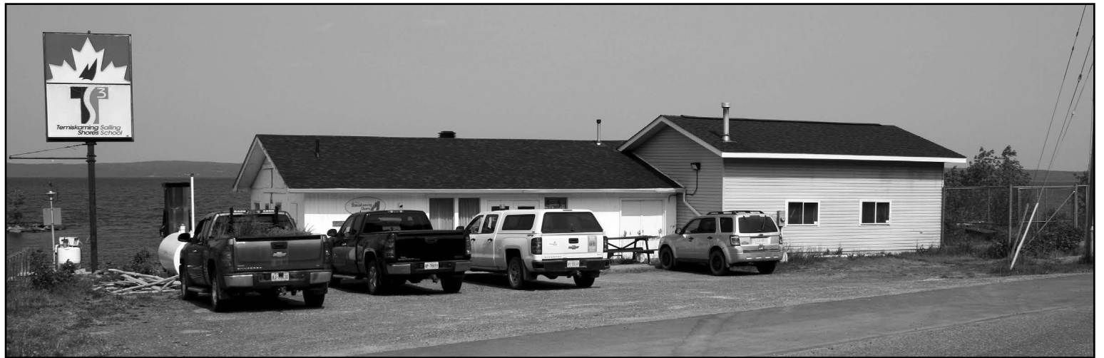
The parks and recreation building south of city hall in Haileybury will become a municipally run impound facility, on at least an interim basis. Temiskaming Shores is preparing for a pilot project that would see the city take over animal control services. (Staff photo by Diane Johnston)
